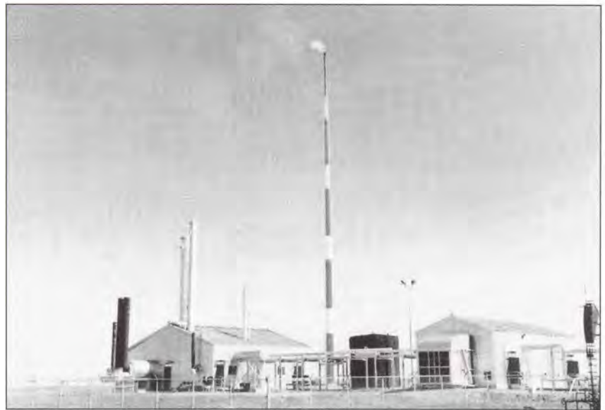
117 GPM Gas Sweetening Plant (also see cover of folder).
